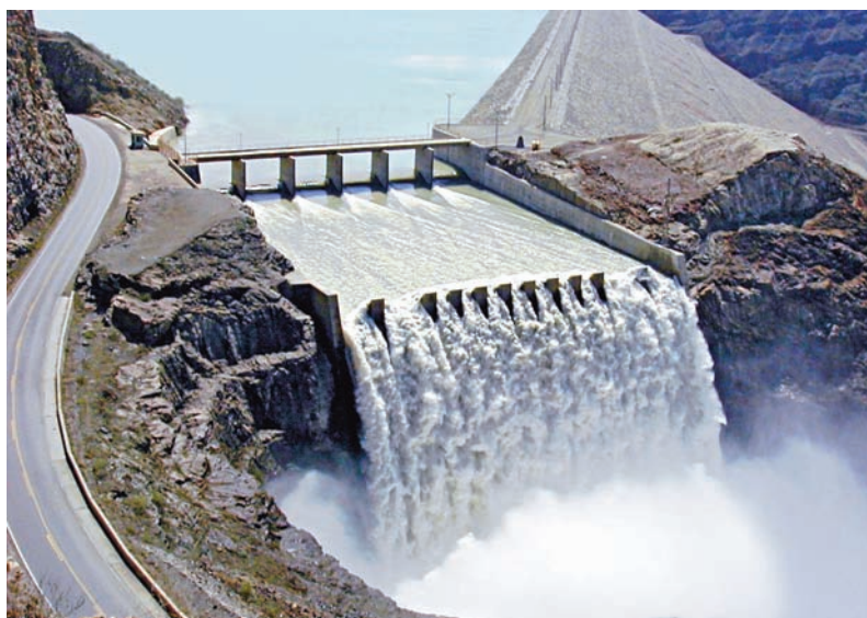
Fig. 6.2. Presa / Dam Gallito Ciego, con aliviadero de demasías operando / with flood spillway under operation.
