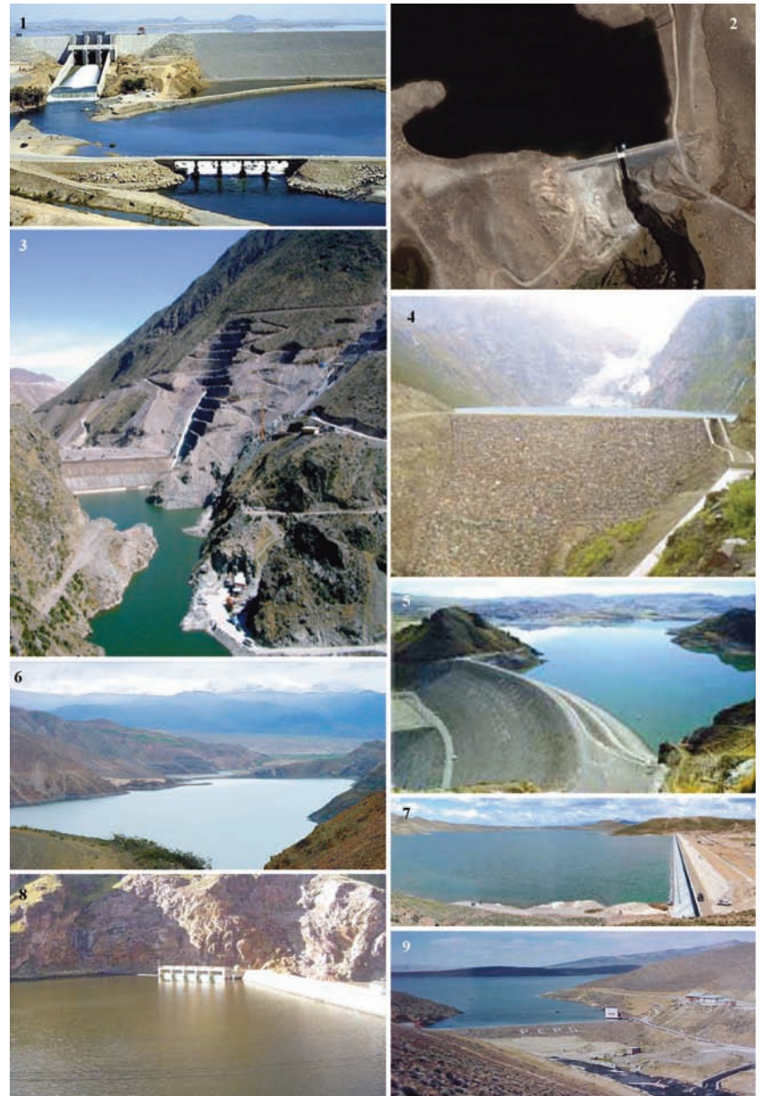
Fig. 11. Presas de tierra y enrocado / Earth (E) - and rockfill dams (R, CFR): [1] Poechos, 1976, E; [2] Huisca Huisca, E; [3] Torata, 2001, CFRD; [4] Rajucolta, 2005, E; [5] Condorama, 1985, R; [6] Aricota, 1962, E; [7] Pillones, 2006, CFRD; [8] Malpaso, 1936, E; [9] Pasto Grande, E. (Fotos fuente / Photos source: Google Earth 2007, Energoprojekt, AUTODEMA, ELECTROANDES, TRANSLEI).
