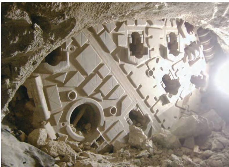
Fig. 17. Punto de entronque de la TBM del túnel Oeste en la caverna de Folledo/Longitudinal section and plan of the connection between the Folledo access adit and the railway tunnels..
