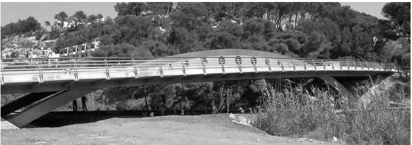
Fig. 6. Vista general del puente/ General view of the bridge.
