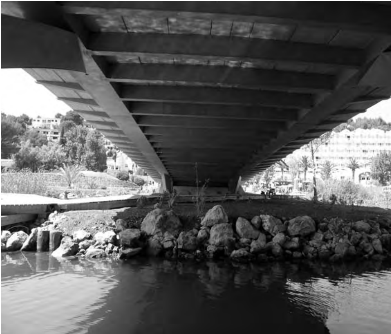
Fig. 5. Vista inferior del puente/ Lower view of the bridge.
