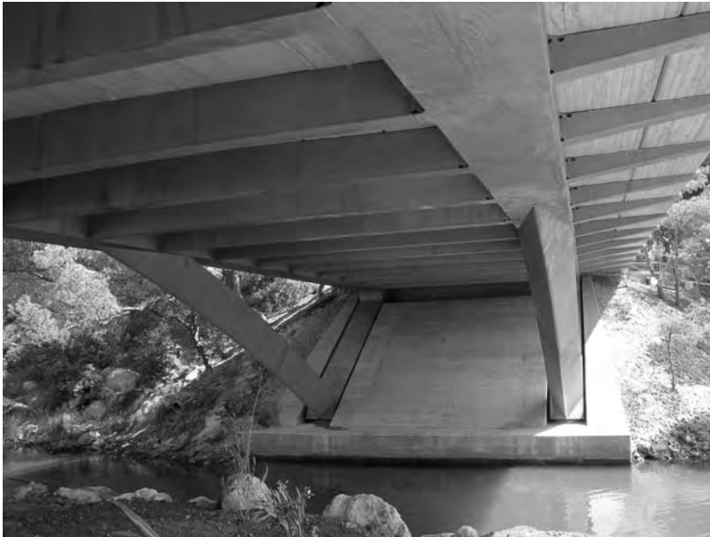
Fig. 3. Estribo 2. Vista de la estructura completa/Abutment 2. View of complete structure.
