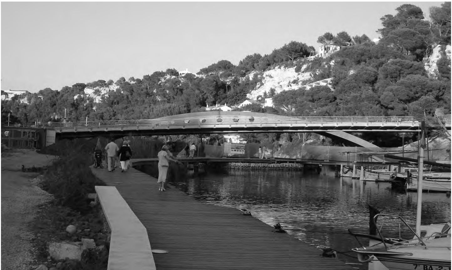
Fig. 17. Estructura finalizada/ Completed structure.
