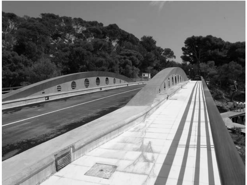
Fig. 10. Vista superior del tablero/ Upper view of the deck.
