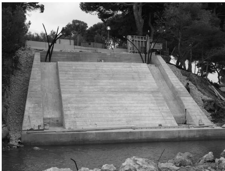
Fig. 2. Estribo 2. Vista durante construcción/ Abutment 2. View during construction.
