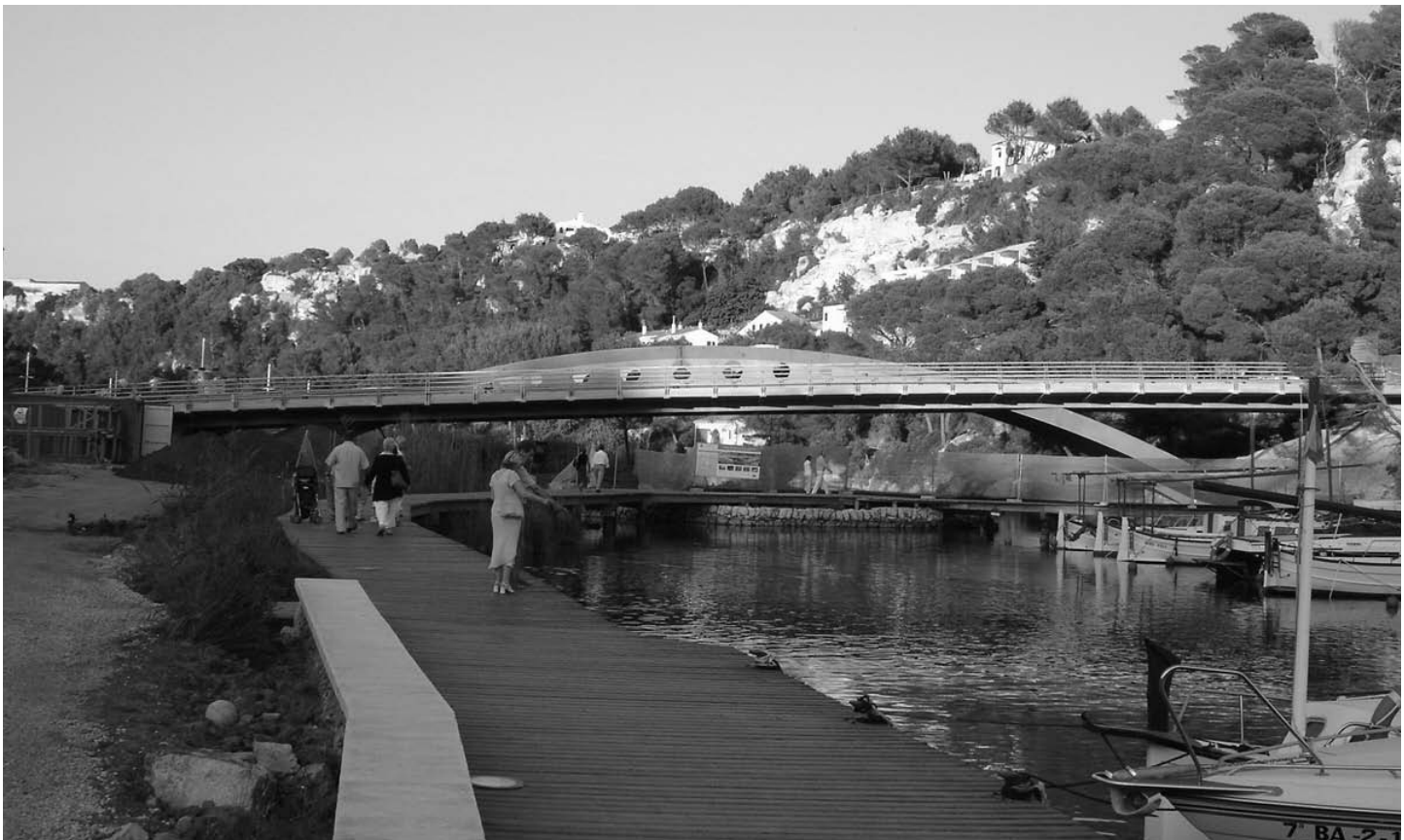
Fig. 17. Estructura finalizada/ Completed structure.
