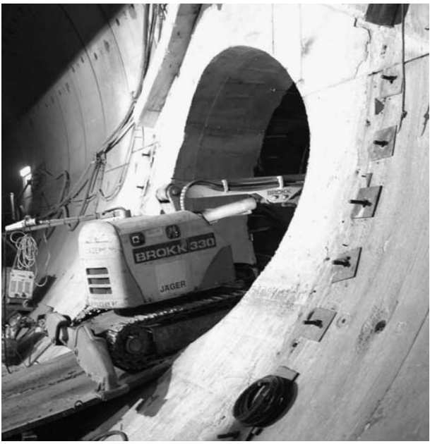
Entronque terminado/Completed junction.
