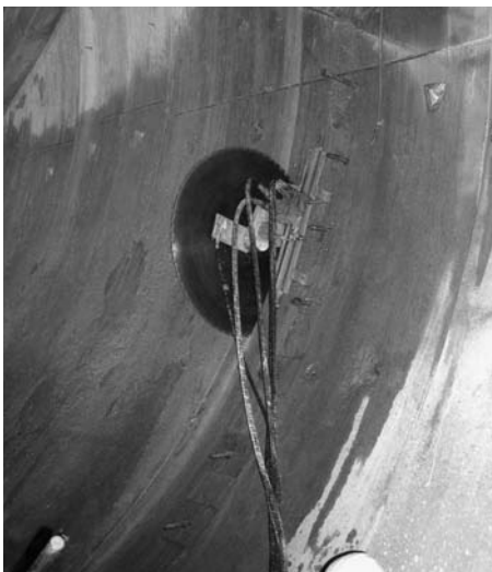
Corte de las dovelas/Cutting of segments.
