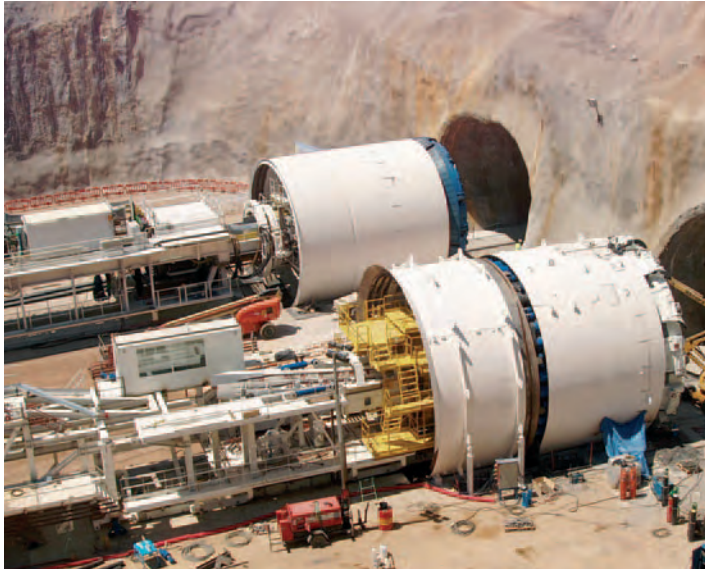
Fig. 7. Tuneladoras del lote 1 de los túneles de Pajares. En primer lugar, simple escudo del fabricante NFM-Wirth. Al fondo, simple escudo de Herrenknecht/TBMs for contract 1 of the Pajares Tunnels. The TBM in the foreground is an NFM-Wirth single shield TBM, while that in the background is a Herrenknecht single shield TBM.
