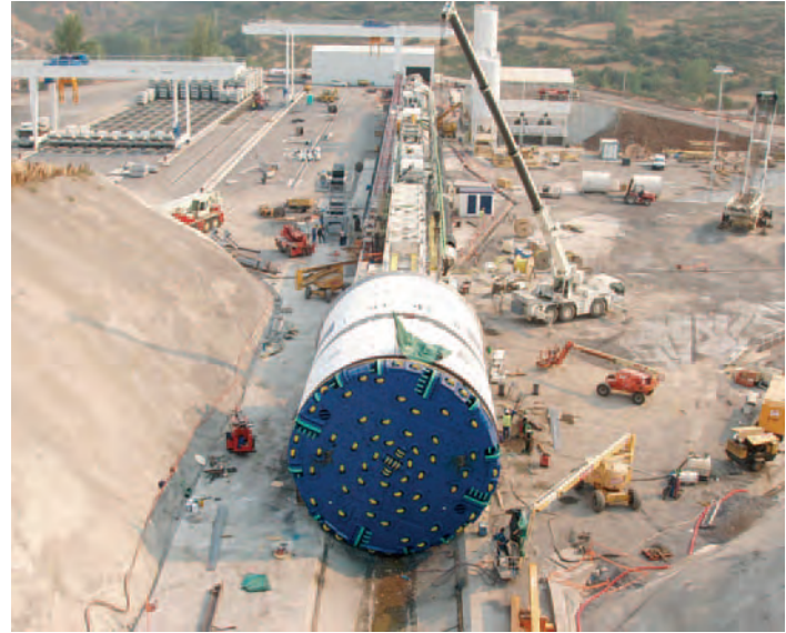
Fig. 7. Tuneladoras del lote 1 de los túneles de Pajares. En primer lugar, simple escudo del fabricante NFM-Wirth. Al fondo, simple escudo de Herrenknecht/TBMs for contract 1 of the Pajares Tunnels. The TBM in the foreground is an NFM-Wirth single shield TBM, while that in the background is a Herrenknecht single shield TBM.
