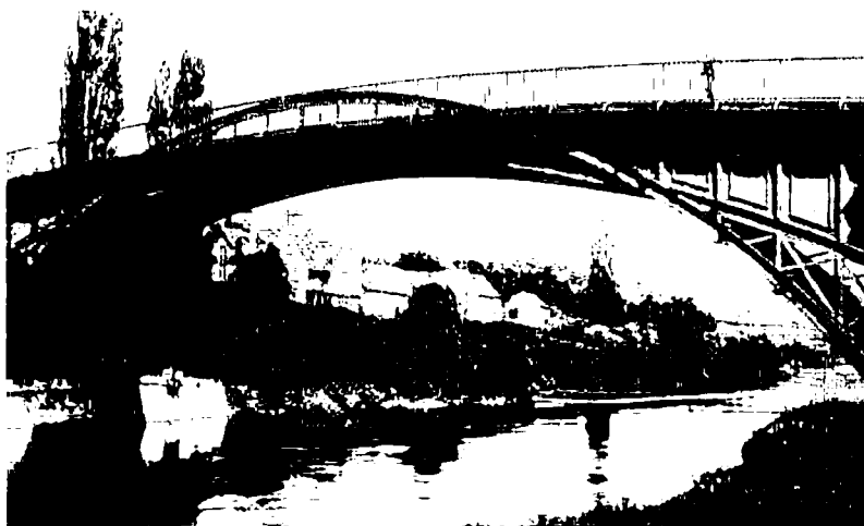
Fig. 7. Buidwas Bridge, Coalbrookdale.
