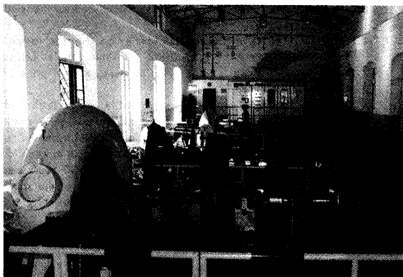
Central de Goizueta, rehabilitada en 1991/ Goizueta Power Station rehabilitated in 1991.
