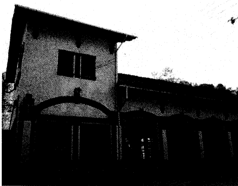
Central de Oroz-Mugaire, rehabilitada en 1992/Oroz-Mugaire Power Station rehabilitated in 1992.
