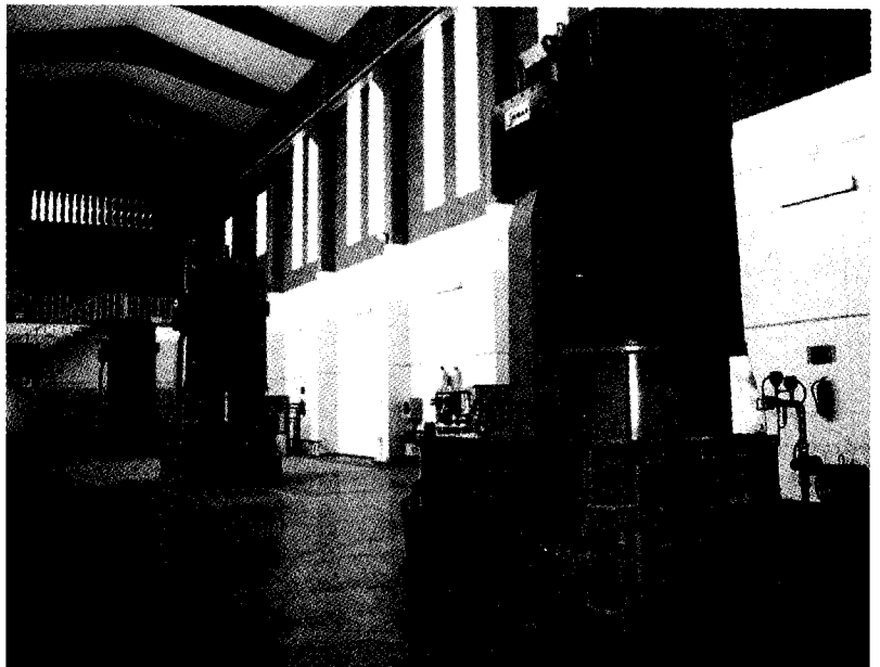
Central de Tudela, vista interior/Interior view of Tudela Power Station.
