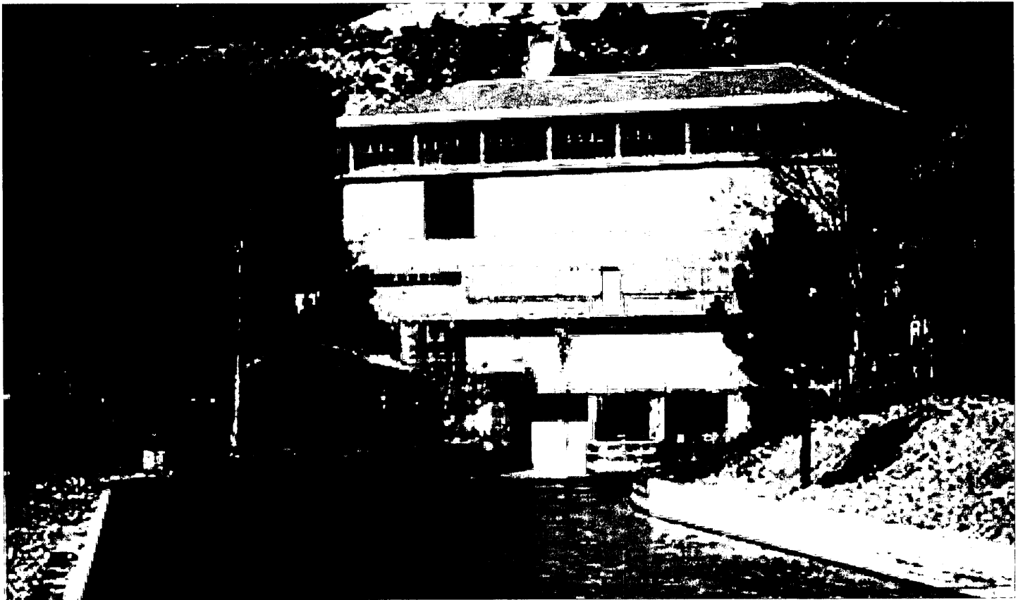
Minicentral Hidráulica/Small Hydraulic Power Plant.
